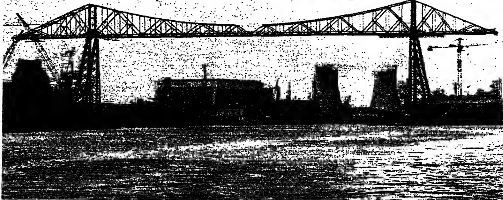
The Transporter Bridge over the river Tees at Middlesbrough
